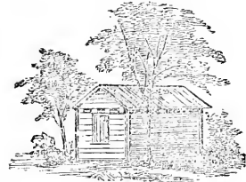
Fig. 1.—Rough or Shanty Ice-House, left open under the eaves for ventilation.
